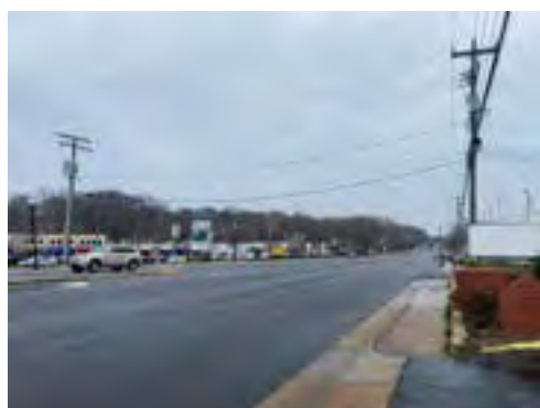
Narrow sidewalks next to wide roads
