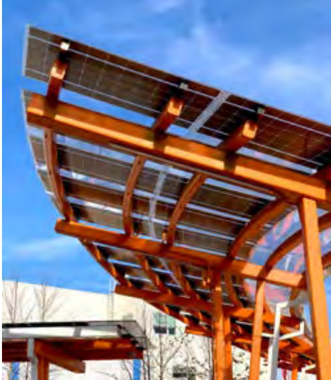
LSX Solar Panel Canopies | https://lumossolar.com/lumos-solar-powered-ev-charging-station/neocity_super-stunner/
